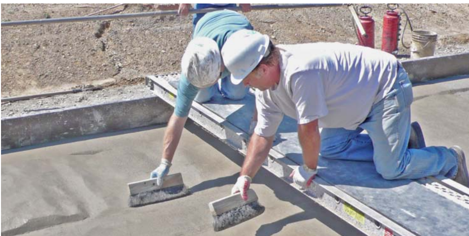
Paved Rough Road Construction
