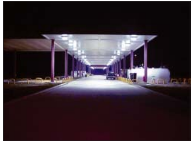
Night view of the new fuel plaza
